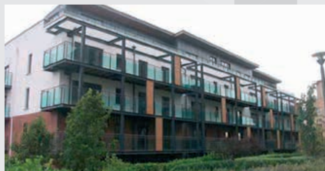
Rathborne | Pelletstown, Dublin 15 Long term lease of 60 apartments to Circle Voluntary Housing Association. 60 units completed and occupied in December 2014 / Q1 2015
